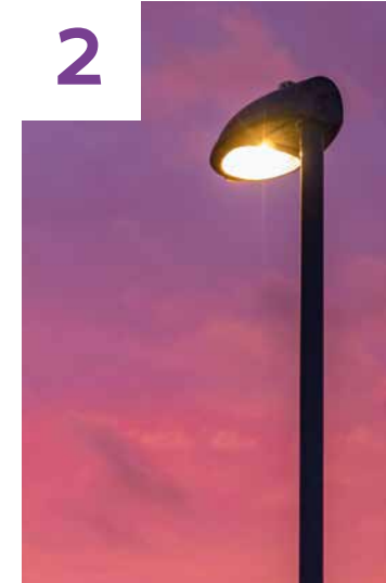
We've contributed to the safety and appearance of the wider neighbourhood by installing more street lighting and repairing 330m of fencing.
